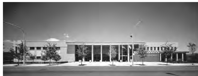
Fig 12. 22nd District Police Station, Chicago, Illinois, 2005.
