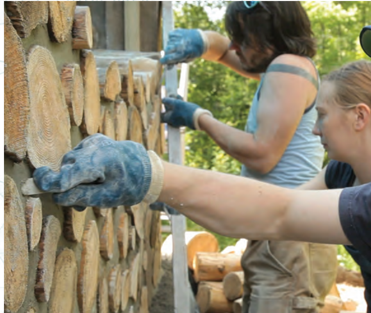
Studio members Schuyler Smith, Claire Halpin, and Todd Zima practice the construction method of wood masonry—a low-carbon, highly thermal method of building that Studio Gang updated to meet twenty-first century criteria for the Arcus Center project.
