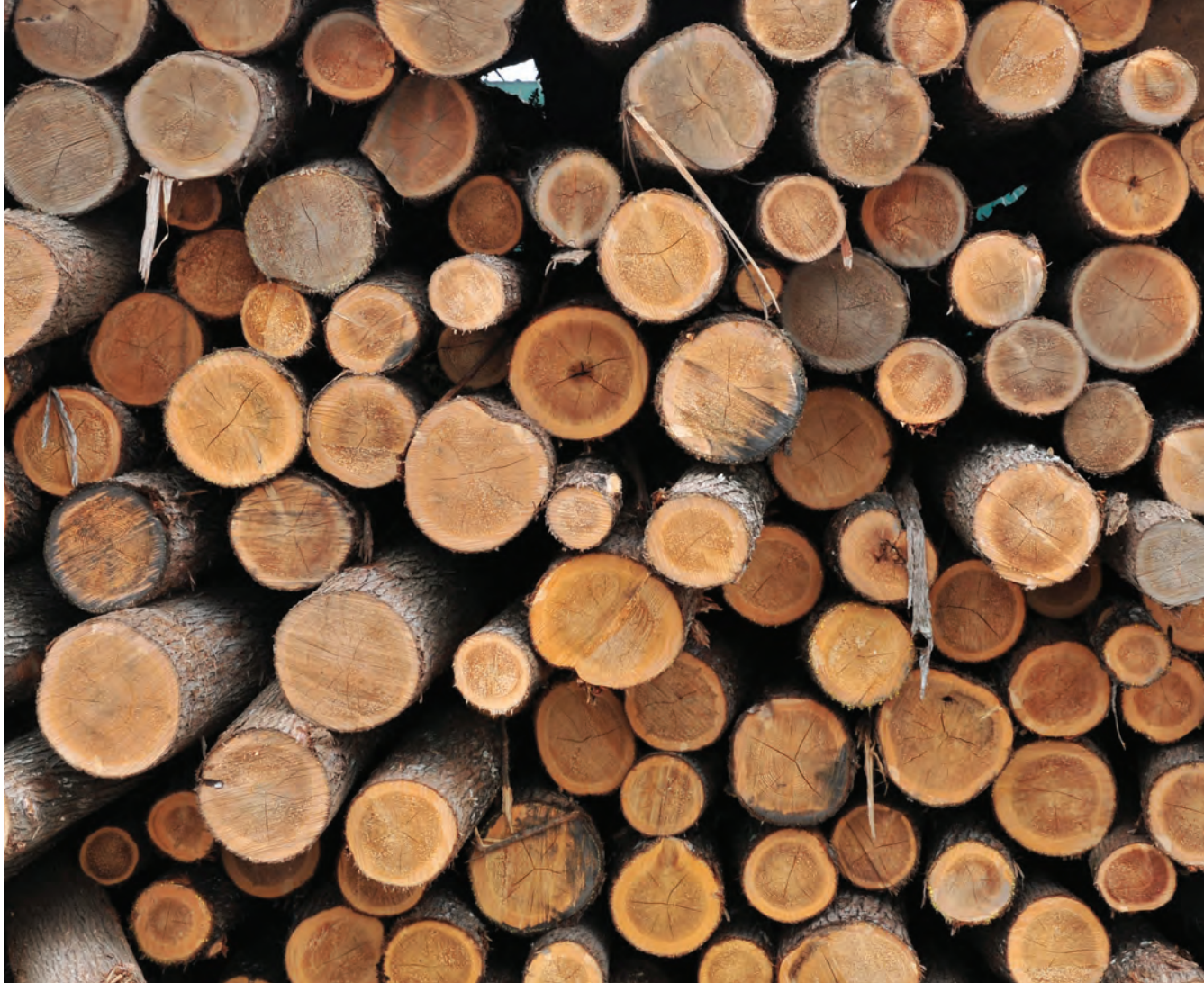
Tree sections of different shapes and sizes—each with its own unique set of growth rings—are assembled together to form the exterior walls of the Center.
